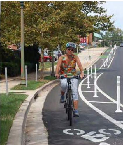
A separated bike lane protected by paint and flex-posts. Image: Montgomery County Planning, Maryland.
