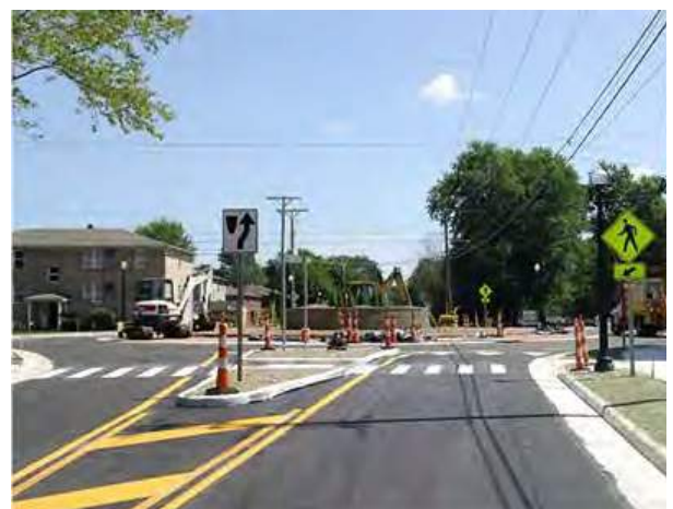
Roundabout at Mathews & Sheridan Rd. Mahoning County
