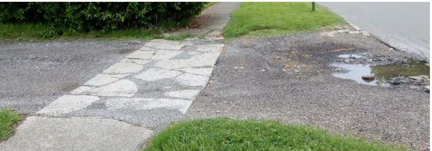
Sidewalk near Stadium Drive Elementary (2018).
